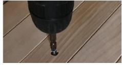
7. Secure the back rest to the back panel using the predrilled holes in the backrest and attach the accessories.
